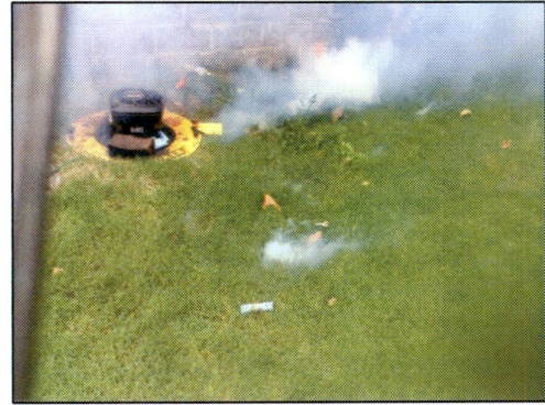
Smoke Testing Defect (RV26)8036-8032
